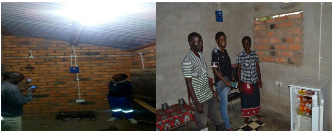
Solar Micro grid project in Sinda district of Eastern Province
